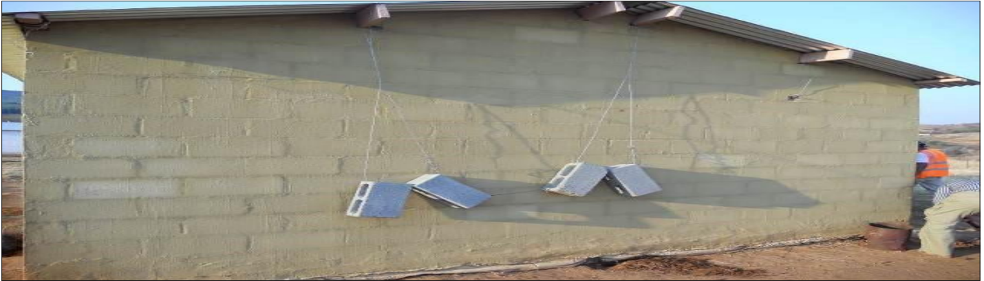
Figure 4 : Typical roof anchoring system used for low-income houses
