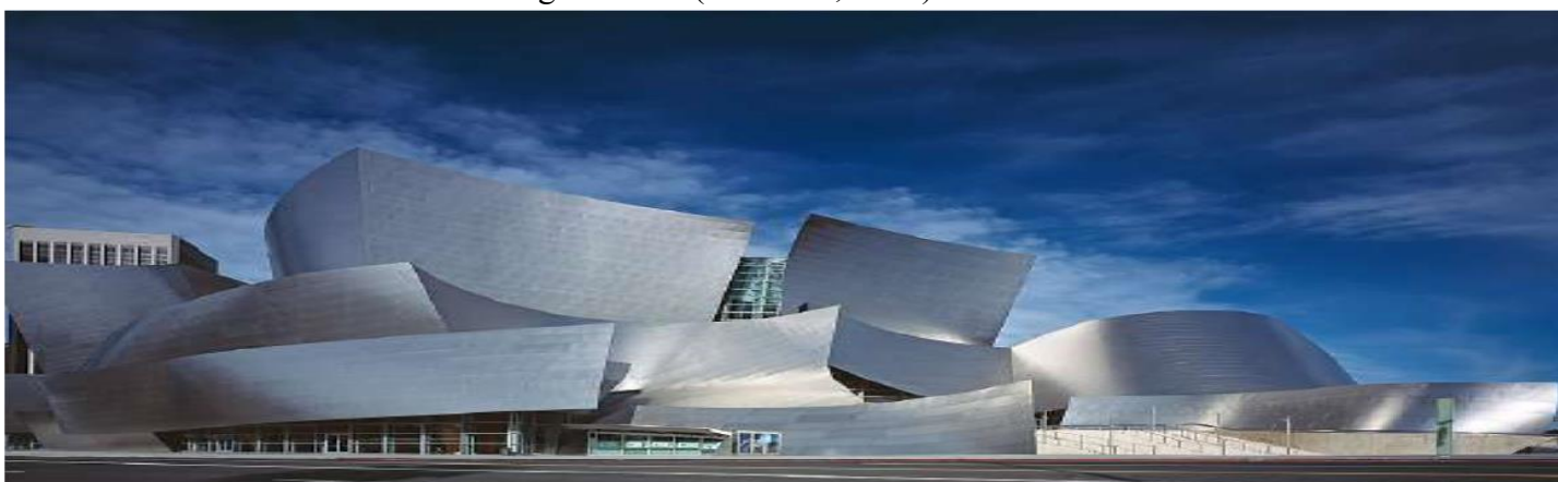
Figure 2: Walt Disney Concert Hall in Los Angeles (2003)
