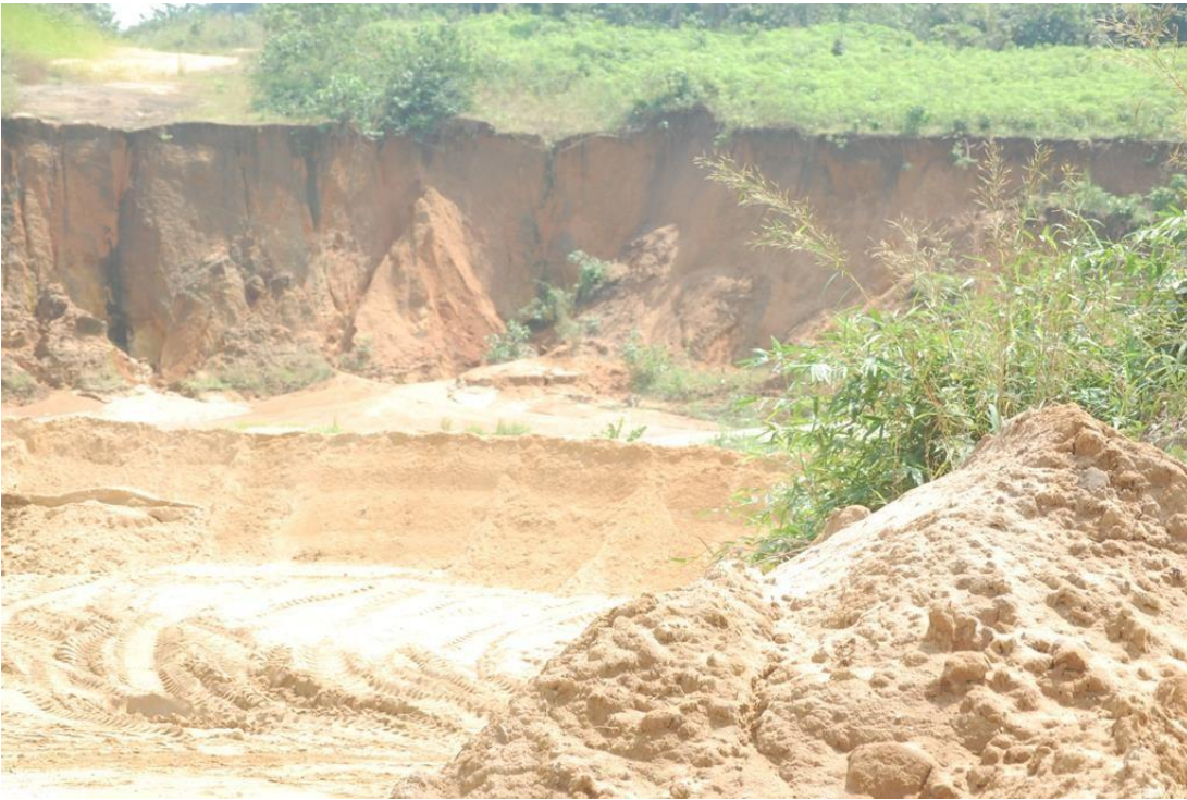
Figure 1: Borrow Pit Source: Field Survey, 2024
