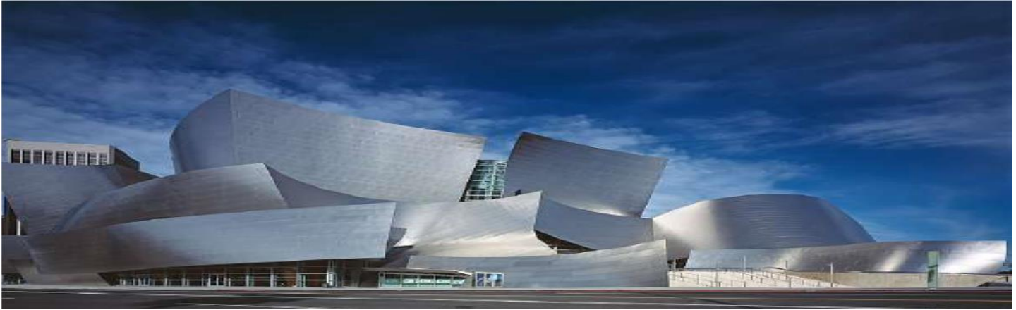
Figure 2: Walt Disney Concert Hall in Los Angeles (2003)
